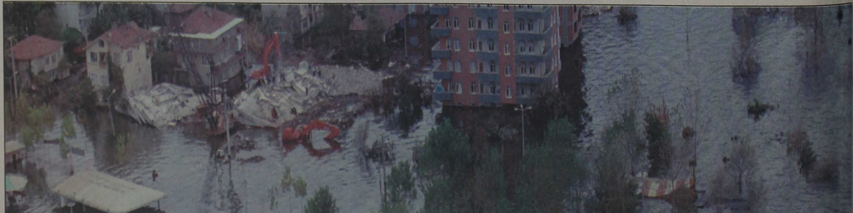
Flooding from a subsequent tidal wave continues to hamper repair operations to earthquake damage near Izmit, Turkey. The three-ship Kearsarge Amphibious Readiness Group is at Izmit to aid v
