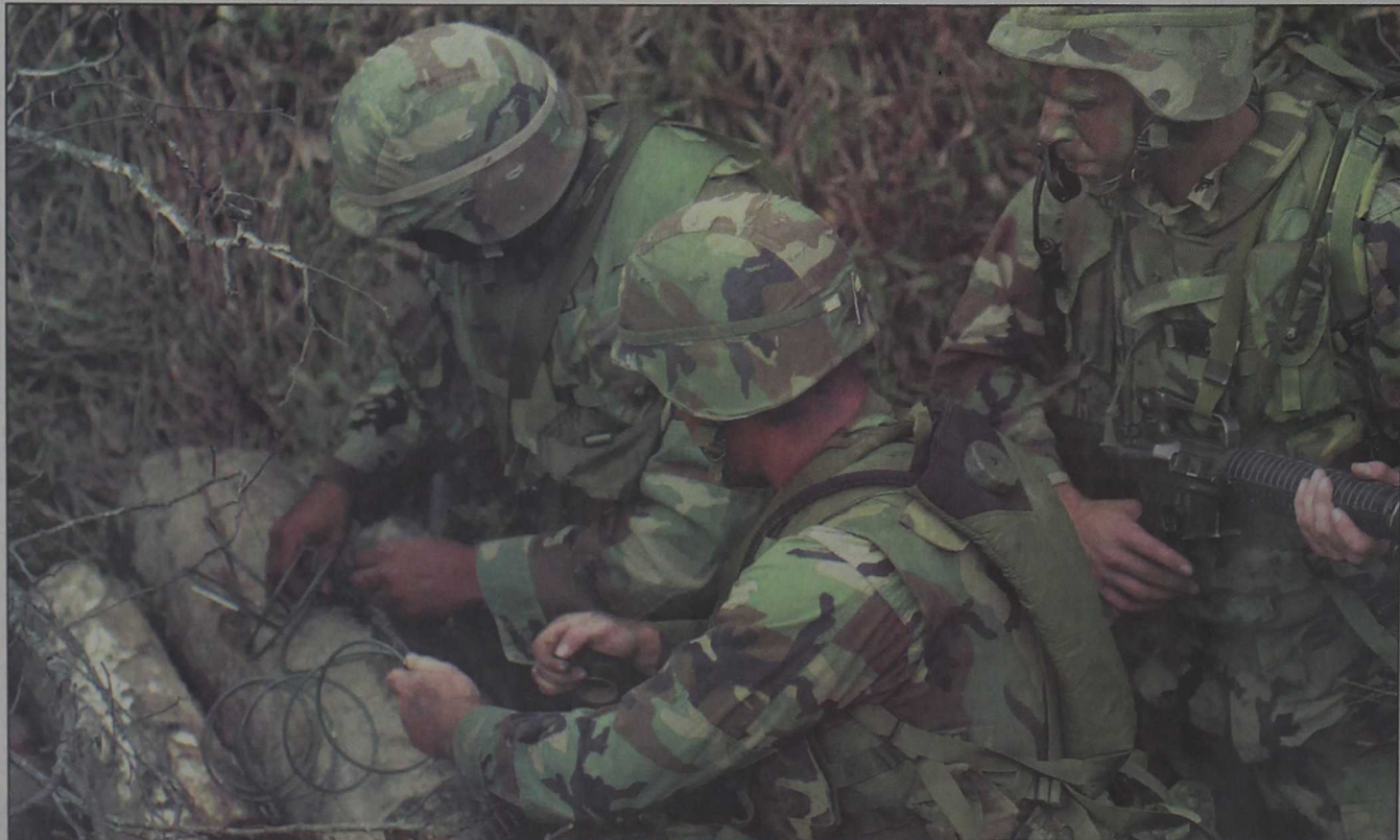
Marines from 2d CEB, set a demolition charge to take out a bridge.
