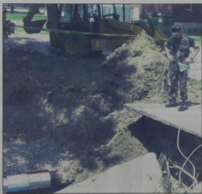
THE BIG SPILL — The 50-year-old water pipe, which burst Wednesday caused Marines living and working on base a major inconvenience. LCpl David Nicholson, commanding officer for Base Maintenance Office examines the pipe, which was fixed in time for an afternoon shower.
