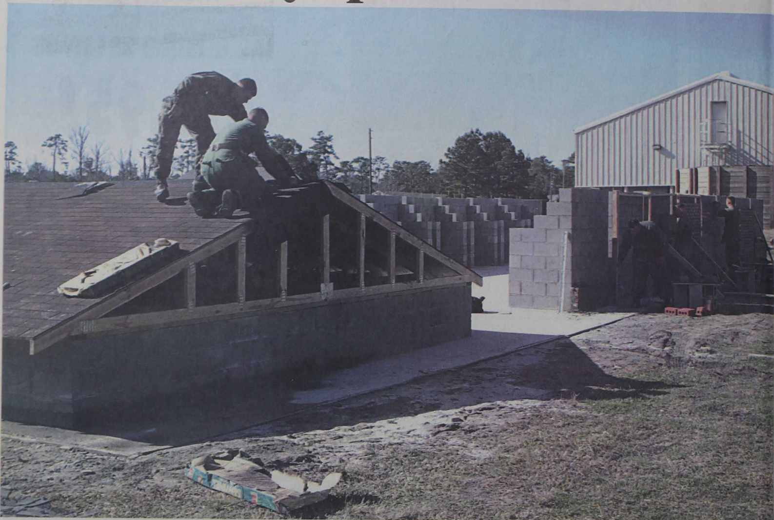
Above, combat engineers build a new breach assault pit for demonstrating how to get through a wall or roof at the SOTG Complex in Stone Bay. Below, MSSG-24 engineers build the roof closer to the ground making access easier for instructors as well as reducing efforts after training.
