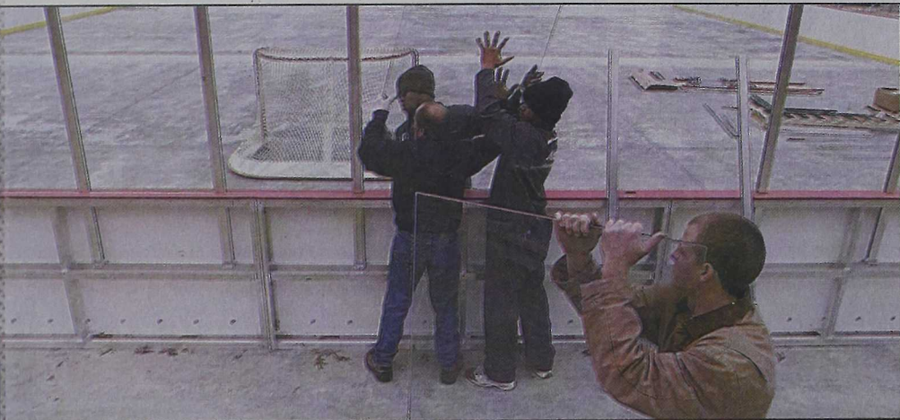
Jason Hoehn steadies a piece of tempered glass while fellow workers Duron Barker, Rod Stidham and Justin Lord place a pane into support panels at the newly constructed professional roller hockey rink.
