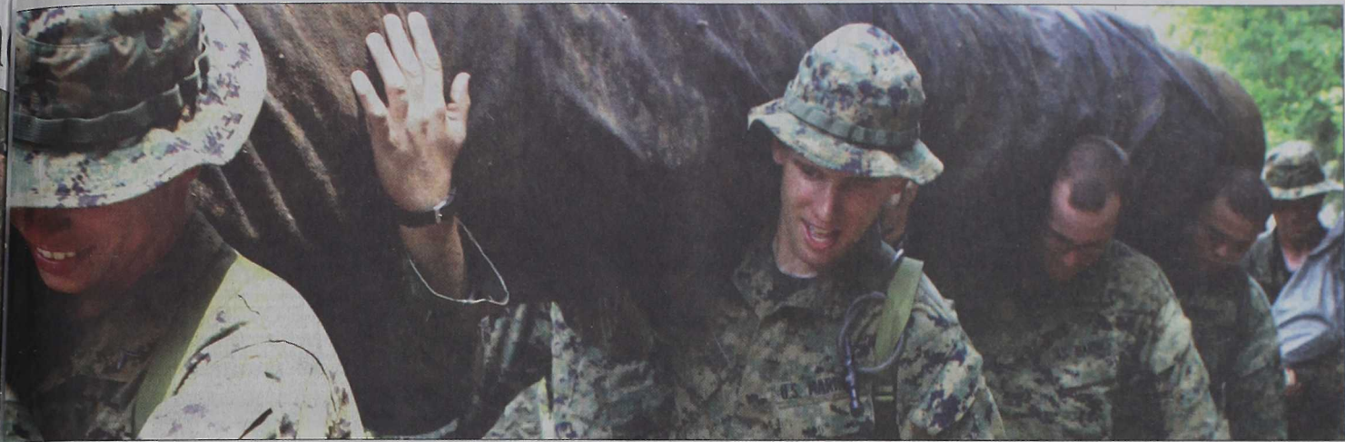
Marines deployed in support of Philippine Interoperability Exercise 2005 carry a roll of Geo-textile matting, a thick, watertight compound that disperses the weight of vehicles traveling over the road so the gravel does not shift easily after prolonged use. The matting is used to build a durable gravel road during a bilateral relations project June 28 to July 16.
