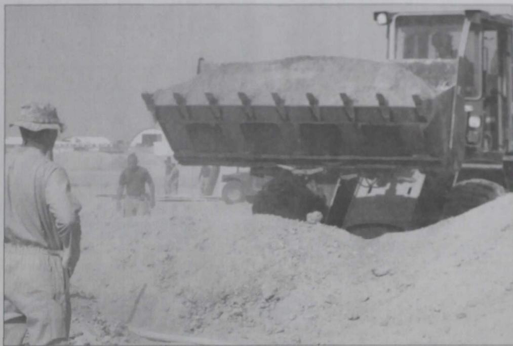
Sergeant Clayton K. Anderson, a Phoenix, native with Bulk Fuel, A Company, 6th Engineer Support Battalion, augmenting 8th ESB in direct support of Combat Logistics Bn. 8, 2d Force Service Support Group (Forward), watches as a CLB-8 front-end loader adds dirt to the berm of a partially-completed fuel pit July 26. The new pits are part of an expansion and renovation project for Camp Fallujah's fuel farm.
