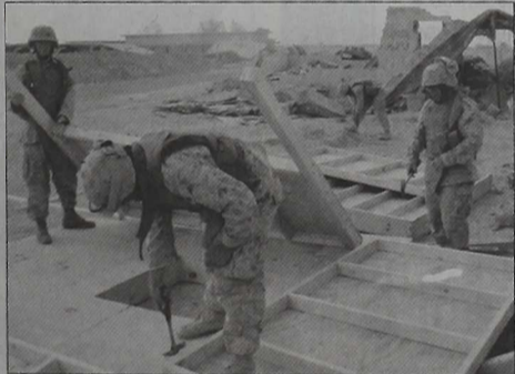
Marines from Equipment Platoon, Combat Logistics Battalion 8, 2nd Force Service Support Group (FWD), work on building a watch tower at the East Fallujah Iraqi Camp near Fallujah, Iraq. The EFIC is used for training new recruits in the Iraqi Army.
