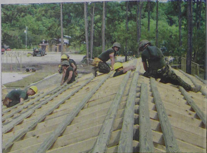
Building huts: Combat Engineers with Company B, 8th Engineer Support Battalion, 2nd Marine Logistics Group, work on a South East Asia hut used at Marine Corps recruit depot, Parris Island.
