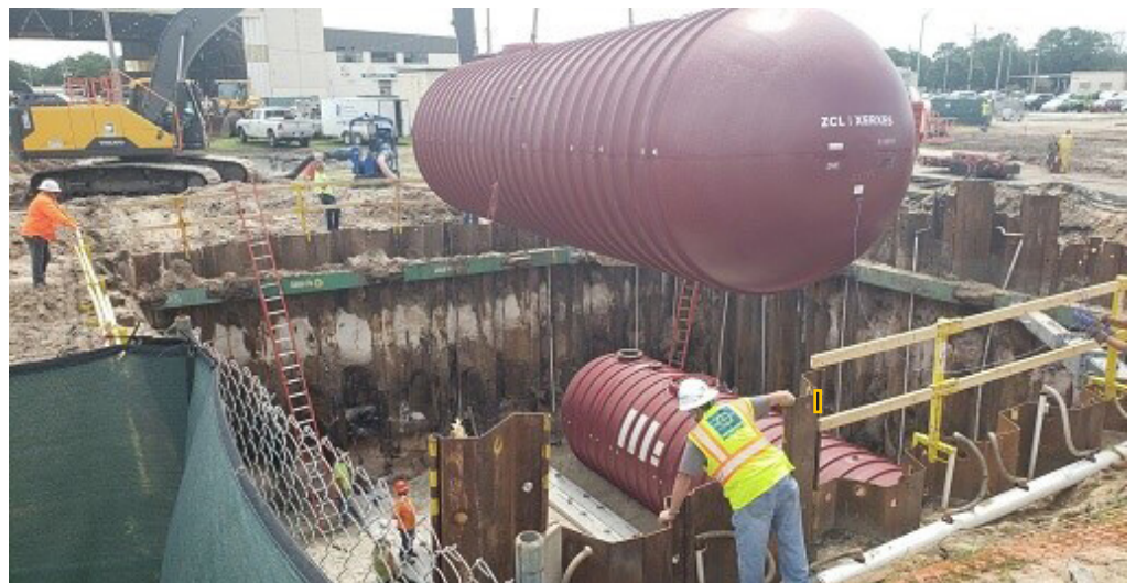
PENSACOLA, Florida 22,000 gallon recovery tanks are installed at Sherman Field in an effort to upgrade fire suppression systems Photo by Michael Ellis.
