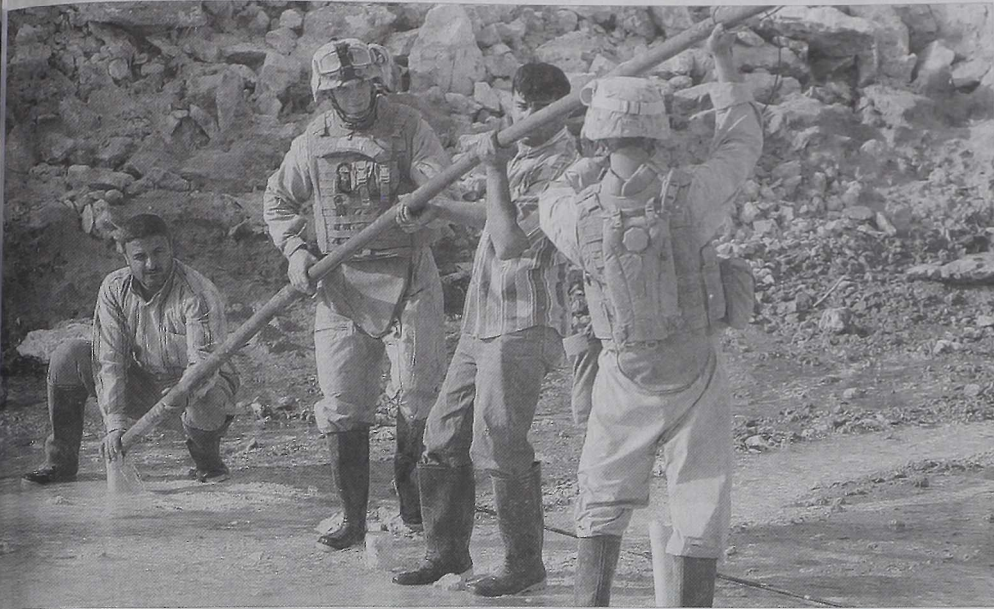
A. White, 23, and Lance Cpl. Dustin D. Sauder, 22, both with Company A, 3rd Combat Engineer Battalion, Regimental Team 5, place four of the 265 Bangalore Torpedoes into pre-drilled holes outside of the Tahadi power plant with the help of two Iraqi contractors. Cpl. Shawn Coolman
