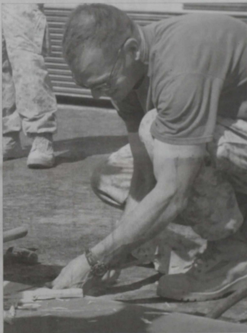
(Above) Marines with MWSS 271, attached to the 24th Marine Expeditionary Unit, NATO International Security Assistance Force, lay down AM2 matting while in Kandahar province, Afghanistan. This AM2 matting will be essential in the support of aircraft while conducting operations in support of NATO. (Right) A Marine with MWSS 271, adds another piece to the 96,000 sq. ft. AM2 matting puzzle on a base in Kandahar province March 19. The matting will be used to land and park aircraft. Cpl. Andrew J. Carlson
