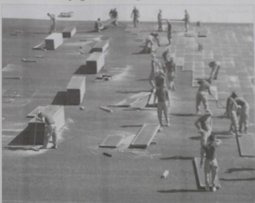
(Above) Marines with MWSS 271, attached to the 24th Marine Expeditionary Unit, NATO International Security Assistance Force, lay down AM2 matting while in Kandahar province, Afghanistan. This AM2 matting will be essential in the support of aircraft while conducting operations in support of NATO. (Right) A Marine with MWSS 271, adds another piece to the 96,000 sq. ft. AM2 matting puzzle on a base in Kandahar province March 19. The matting will be used to land and park aircraft. Cpl. Andrew J. Carlson
