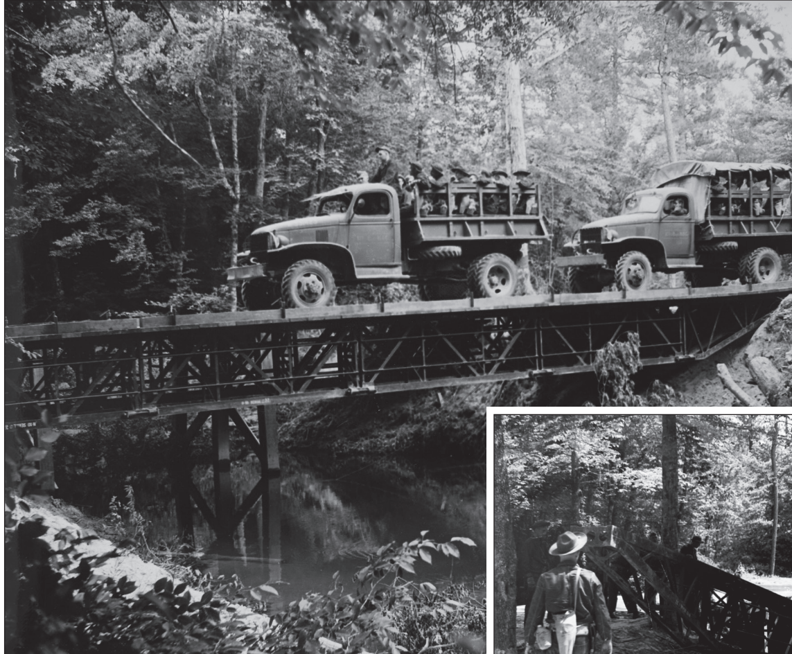
At right, engineers from the 32nd Division's Company A, 107th Engineers pull a steel truss for a 72-foot bridge weighing up to 15 tons at Camp Livingston, La., May 23, 1941. U.S. Army Signal Corps photos
