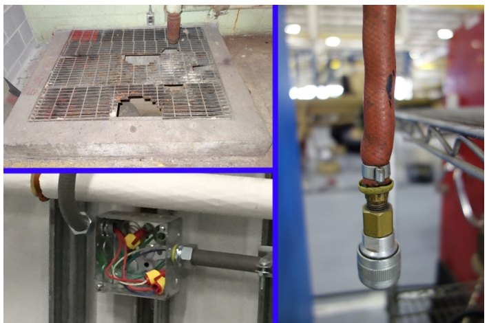
Examples of potential safety hazards that should be reported using the Hazard Reporting Process.
