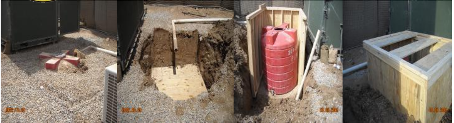
Above: Steps leading to an installed, in-ground water tank. The tank now provides running water to a CF Patrol Base in Northern Iraq.
