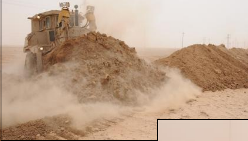
Clockwise from Top, Left: The D9 pushes another huge mound to form the berm; Iraqi Jinood get ready to start up their bucket loader; the Iraqi bucket loader peeks out from behind the berm; 2LT Oney, 1SG Hurlocker and Huda the Interpreter speak with the 4th LA OIC.
