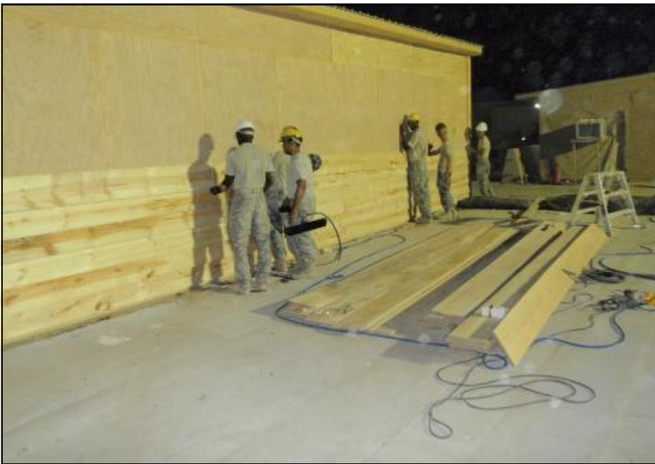
Above: Members of 2/C/84 work on the back of the building and apply the 1"×12"×16' full board siding at night; Right: SPC Alvarez and SPC Brown run the nail gun to speed up the siding process. Although the wood was brittle, the nail gun worked better than expected.
