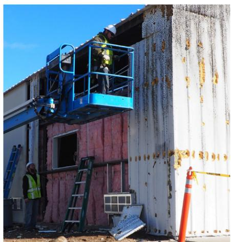
The FHL Logistics Readiness Center and several other buildings are undergoing an exterior facelift (also known as skinning) to replace the woodpecker-damaged wall. The new desert beige color blends in with other newer buildings and helps with energy efficiency. According to the installation Master Plan, buildings are updated every year to meet building requirements.
