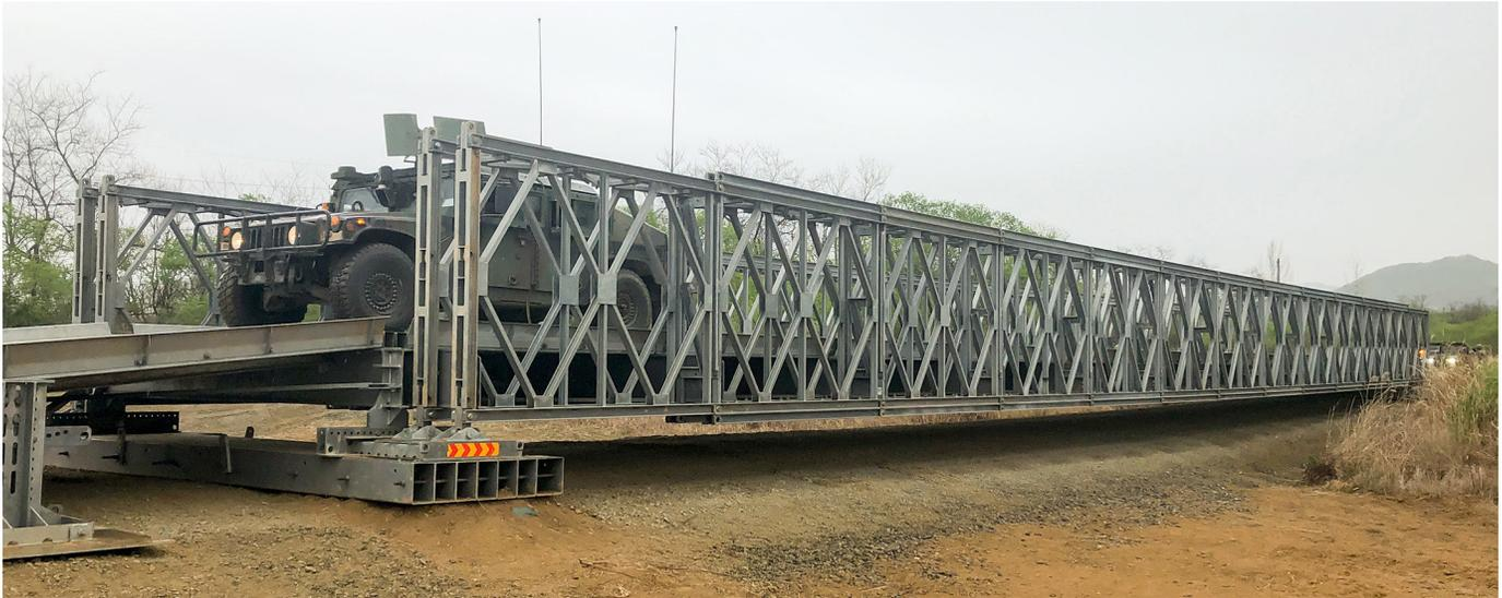
**Figure 3.** A humvee from 3/1 ABCT crosses a 40-meter LSB over a dry gap constructed by members of 814<sup>th</sup> MRBC. (U.S. Army photo by LTC Robert Dion)
