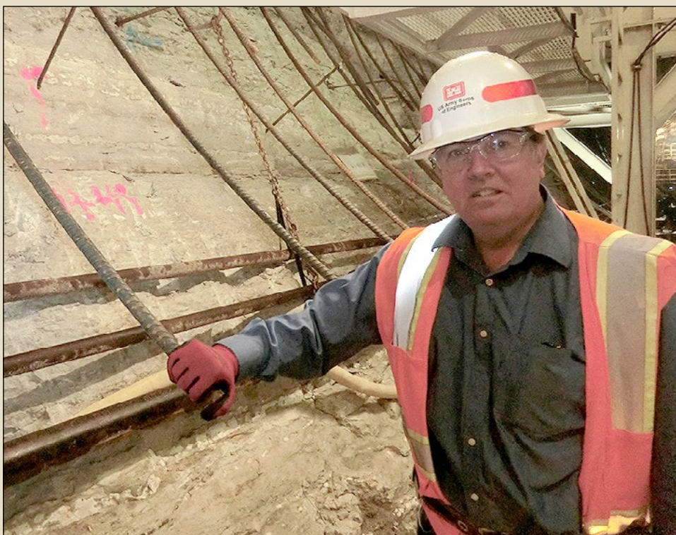
Joe Kissane, a senior geologist with USACE, Chicago District, inspects the foundation to ensure the stability of the McCook Reservoir's main tunnel connection.
