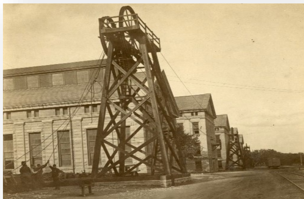
A view of the towers that supplied telodynamic power to the stone shops south of Rodman Avenue (Arsenal Row).
