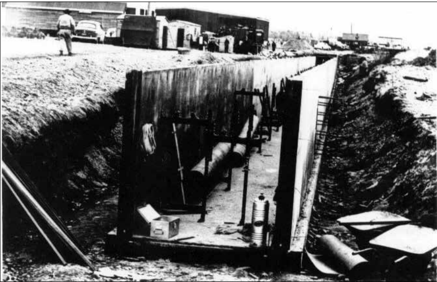
Ladd Field's design included heated utility corridors or utilidors. These concrete tunnels kept pipes from freezing and served as underground walkways connecting residences and work areas. The heat transferred through their lids also served to keep the above ground walkways snow and ice free throughout the long winters. The utilidors were quite a novelty. One 1940s visitor remarked in a bit of an exaggeration that at Ladd, "you do everything underground, and don't come up except to fly." (File photo, Cultural Resources Program)
