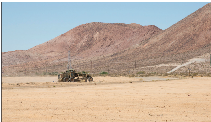
A road grading machine with a 7th ESB Marine behind the controls does its dusty work leveling 20 acres of desert land outside the fenceline behind the Mounted Color Guard stables on the Yermo Annex of Marine Corps Logistics Base Barstow, Aug. 19, 2019. The land is intended for use as a bivouac area for visiting Marine Corps units engaged in training.
