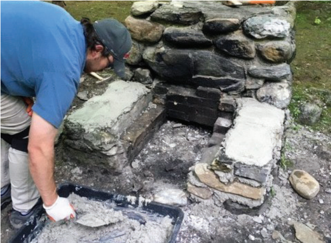
Ethan Bean, Baltimore District archaeologist, applies a mortar wash to the arms of a stone fireplace in Smuggler’s Notch State Park, Vermont, June 2019. (Courtesy photo)
