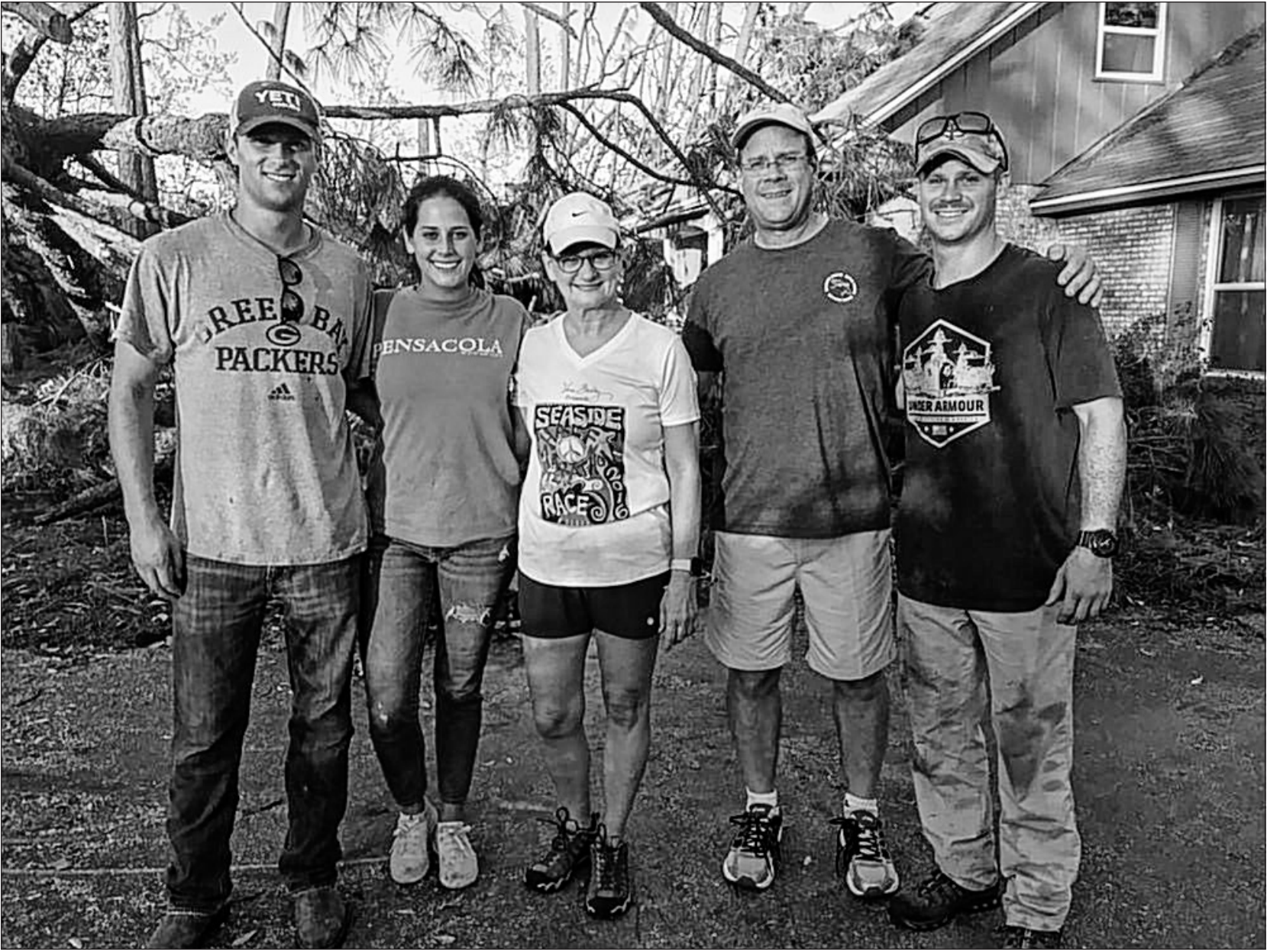
Ensign Andrew Kittel, Carolyn Gadboys, Lisa Churchwell, Gary Churchwell, and Ensign Nicholas Sholty gather after a day of work removing debris, furniture, and carpet from the Churchwell home following Hurricane Michael’s destruction. Ensigns Kittel and Sholty, both student aviators from the “Red Knights” of Training Squadron THREE and Gadboys worked several 14-16 hour days providing assistance to nearly 100 people.
