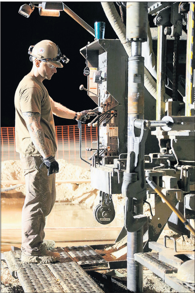
Staff Sgt. Kalie Frantz U.S. Navy Construction Mechanic 1st Class Aaron Wymore, assigned to Naval Mobile Construction Battalion (NMCB) 133, circulates drilling fluid at the bottom of the bore hole and waits for cuttings to come out during water well drilling exploration operations in Riohacha, Colombia, Sept. 1, 2018 as part of Southern Partnership Station 2018. Southern Partnership Station is a U.S. Southern Command-sponsored and U.S. Naval Forces Southern Command/U.S. 4th Fleet-conducted annual deployment focused on subject matter expert exchanges and building partner capacity in a variety of disciplines including medicine, construction and dive operations in the Caribbean, Central and South America.
