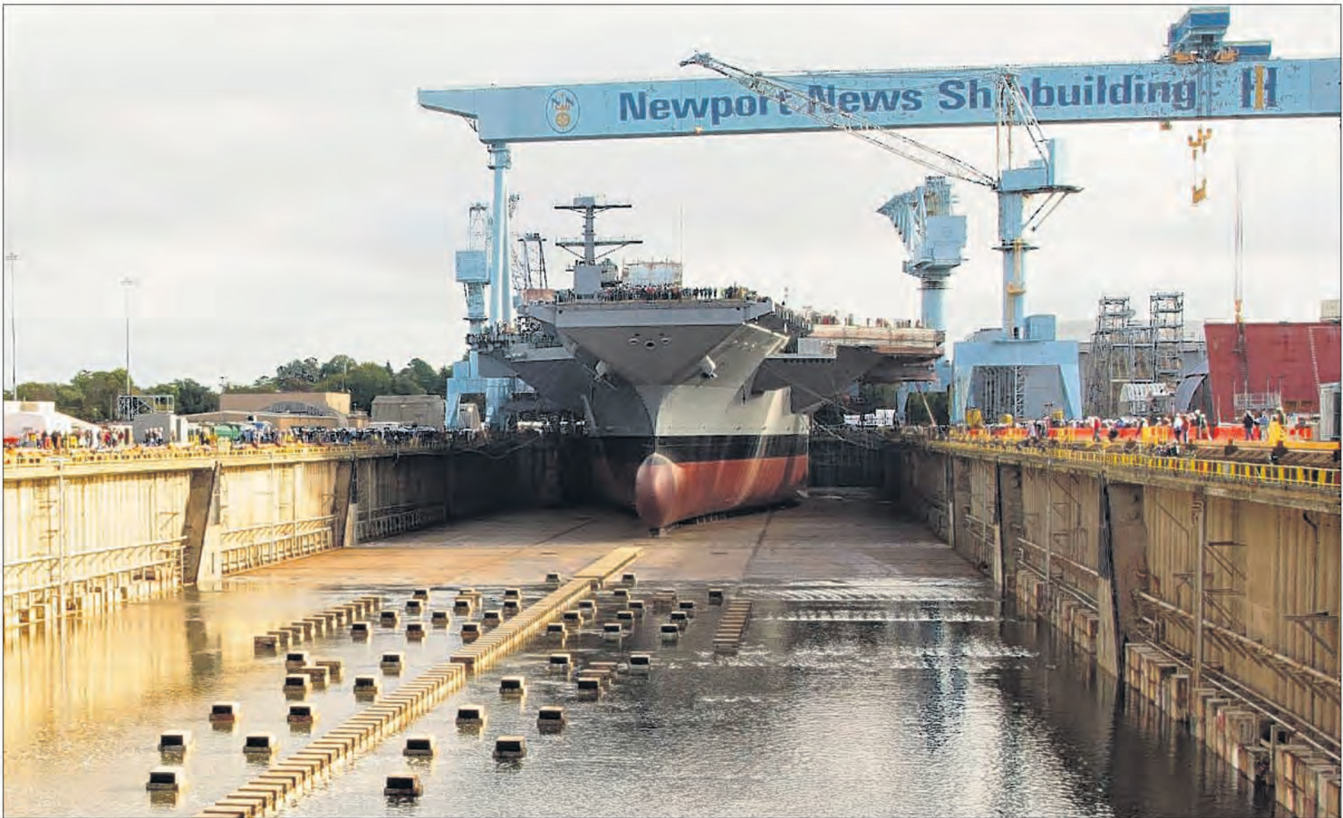
MC3 Adam Ferrero Pre-Commissioning Unit (PCU) John F. Kennedy (CVN 79) reaches another milestone in its construction as their dry dock area is flooded three months ahead of its slated production schedule leading up to the christening of the second Ford-class aircraft carrier, scheduled for Dec. 7. The flooding of the dry dock follows other milestones, including the laying of the ship's keel on Aug. 22, 2015, the placement of the 588-metric ton island superstructure on May 29, and the arrival of the crew on Oct. 1. Kennedy is currently under construction at Huntington Ingalls Industries-Newport News Shipbuilding.
