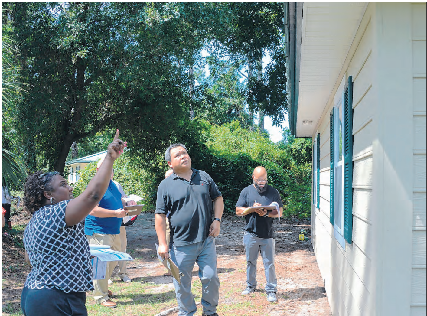
MC2 Nick Grim Student inspectors examine the exterior of a cottage for structural damage or deficiencies as part of their Certified Navy Housing Inspector Level 1 certification at Naval Air Station (NAS) Jacksonville, Sept. 26.
