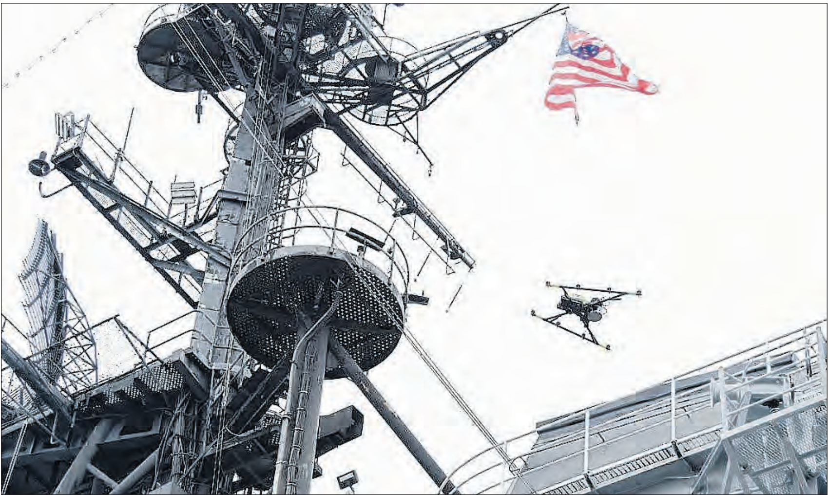
Aboard the USS Midway Museum in San Diego, California, the Office of Naval Research Global (ONRG) TechSolutions held a demonstration of Topside Drone, a corrosion/anomaly detection sensor payload and processing scheme outfitted to a commercial-off-the-shelf unmanned aerial vehicle. Bobby Cummings
