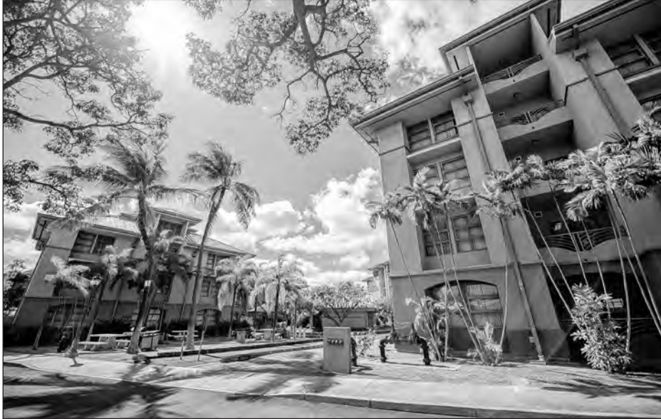
MC2 Charles Oki Gabrunas Hall unaccompanied housing on Joint Base Pearl Harbor-Hickam.
