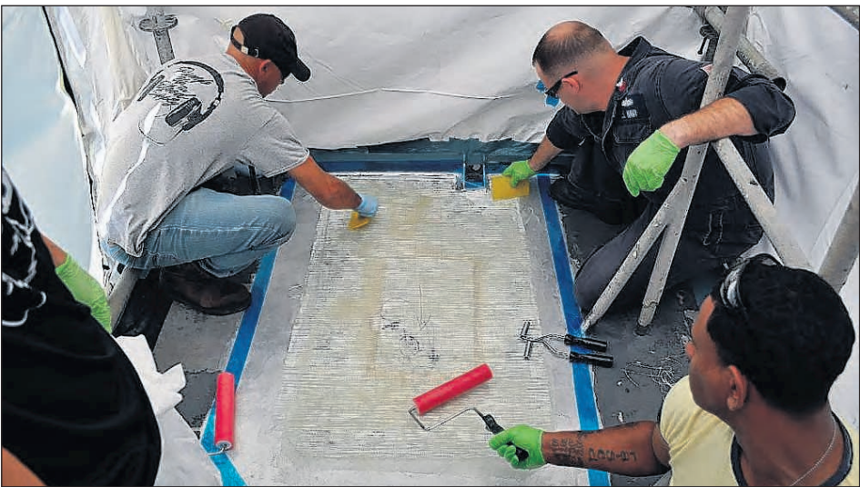
Provided by Dan Hart Regional Maintenance Center team members (clockwise from left) David Marx, Hull Maintenance Technician 1st Class James Falkner and Hull Maintenance Technician 1st Class Desmond Rapach laminate a composite patch on USS Port Royal (CG 73) in January 2019.
