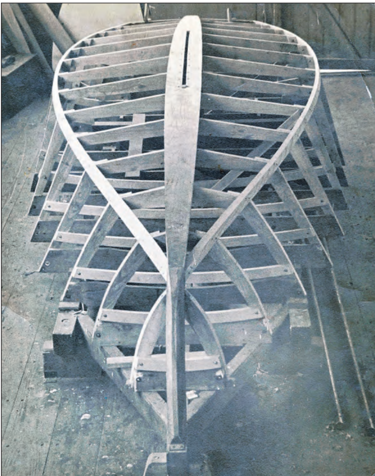
Photo courtesy of Vincent J. Serio, III Hampton One-Design hull under construction on a hull jig. Serio used jigs, patterns and forms to produce and assemble highly accurate parts for the boats. The jig will be on exhibit.
