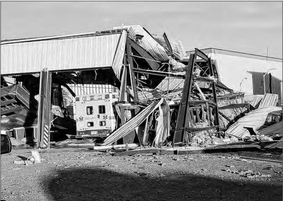
Staff Sgt. Ryan Conroy Hurricane Michael made landfall as a catastrophic Category 4 close to Tyndall Air Force Base, Florida, in the afternoon of Oct. 10. The storm created significant structural damage to the majority of the base and surrounding areas.
