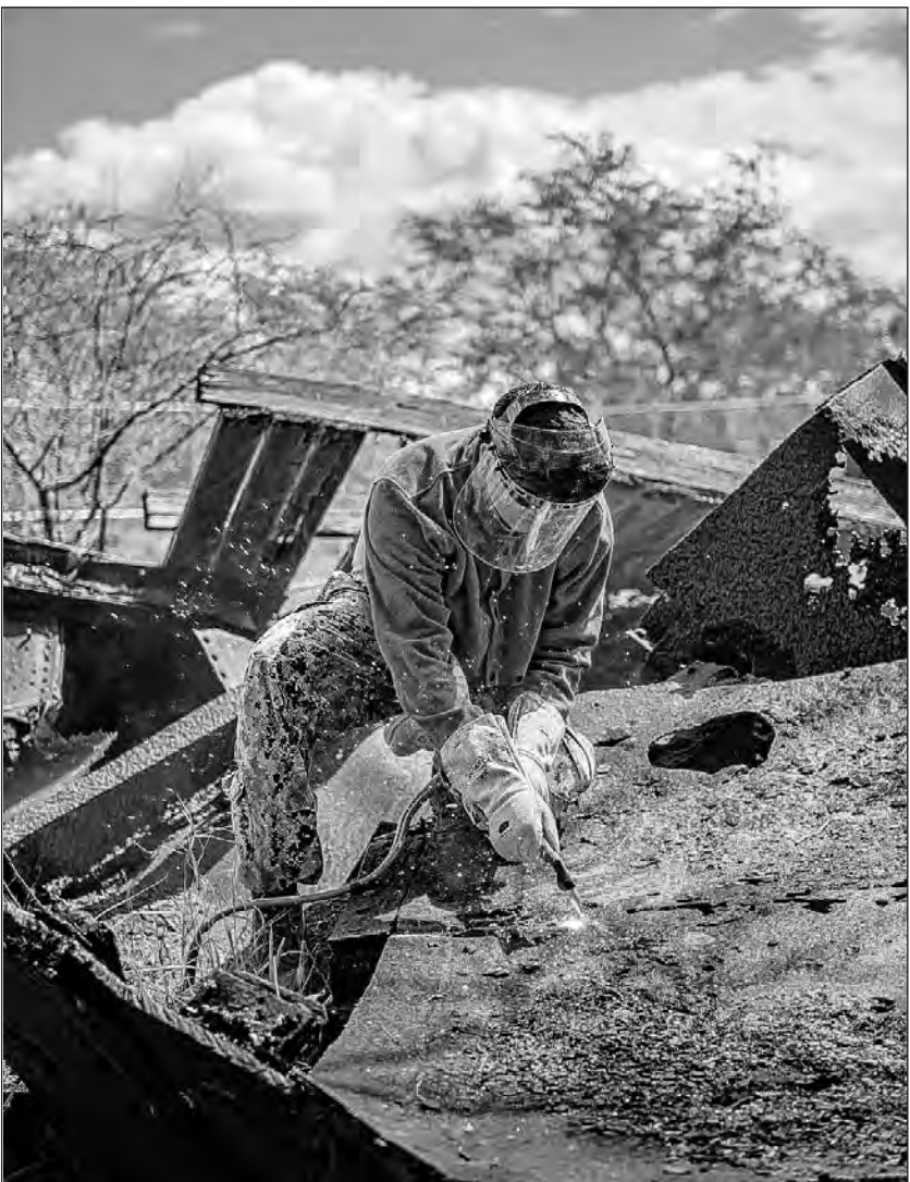
MC2 Allen Michael McNair Steelworker 3rd Class Cameron Fields, crew leader at Construction Battalion Maintenance Unit 303 detachment Hawaii, cuts a piece of steel salvaged from the USS Arizona. This piece, as well as other historical relics, will be displayed in one of more than 100 locations around the world. These visible pieces will allow the public to consider and discuss the significance of the December 7, 1941 attack on Pearl Harbor and World War II.
