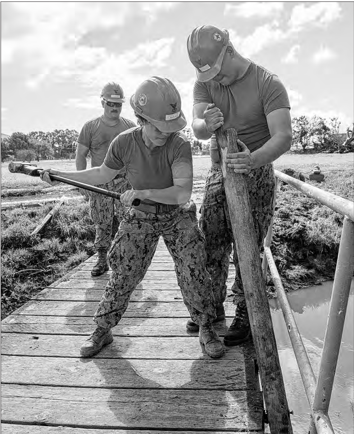
Steelworker 2nd Class Morgan Klaus, left, from Weston, Florida assigned to Naval Mobile Construction Battalion (NMCB) 5, removes old support beams during a bridge reconstruction project on Marine Corps Base Camp Pendleton, California. The new bridge will connect the I Marine Expeditionary Force and NMCB-5 camps giving them the ability to conduct military base construction and maintenance in a joint environment in support of Pacific Blitz 2019 (PB19). Working hand-in-hand, the Navy expeditionary force and Marine Logistics Group capabilities complement each other in the building of advanced naval bases. PB19 provides realistic, relevant training necessary for an effective global U.S Navy and Marine Corps.
