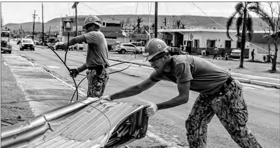
MCC Matthew R. White Seabees assigned to Naval Mobile Construction Battalion (NMCB) 1 remove debris from a road during recovery operations following Typhoon Yutu.
