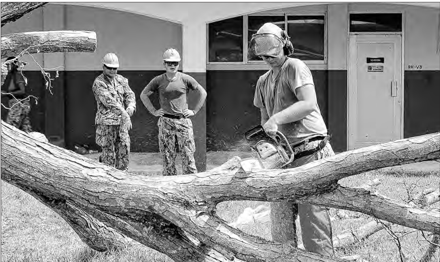
Gunnery Sgt. T. T. Parish Construction Electrician 3rd Class David Yoder, assigned to Naval Mobile Construction Battalion (NMCB) 1, cuts a downed tree with a chainsaw at the junior senior high school in Tinian, Commonwealth of the Northern Mariana Islands, Oct. 31, 2018.
