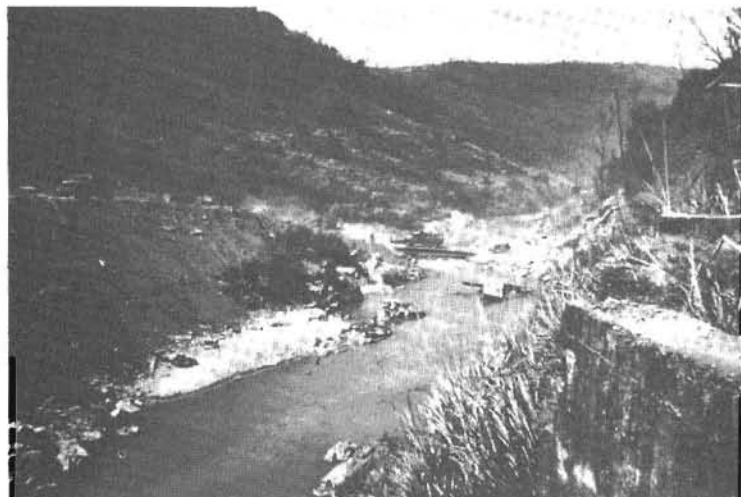
The abutment in the right foreground was all that remained of the bridge across the Quan Tri River.
