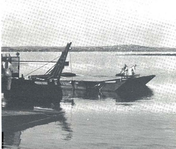
Once fully extended in the water, the sections are linked together as required. Engineers preparing for retrieval of the Ribbon Bridge section.
