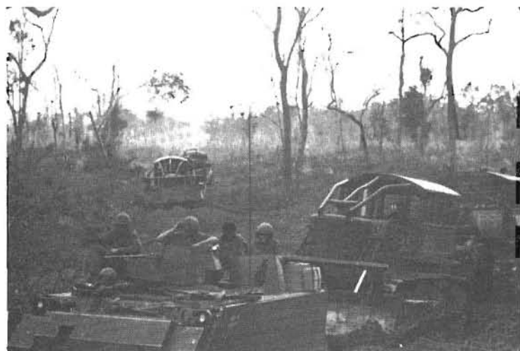
Engineers "Clearing the Way".
