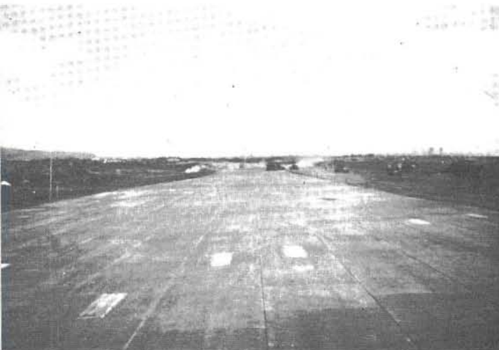
The main airstrip at Khe Sanh overlayed with MX-19 matting.
