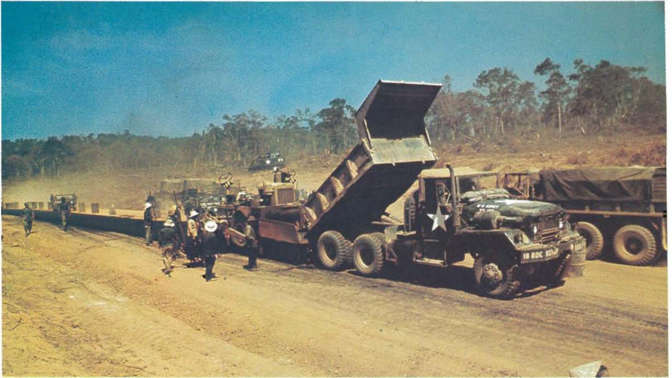
Highway 19 is surfaced with asphalt.
