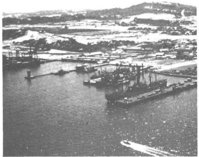
Ships have no problem unloading cargo here at Cam Rahn Bay. Engineers built the four deep draft piers.
