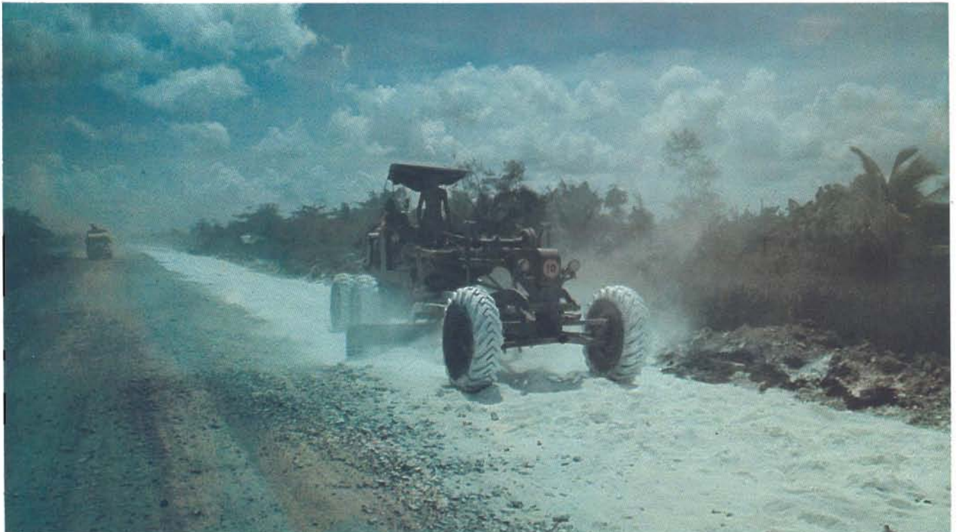
Grader is used to spread and level lime.
