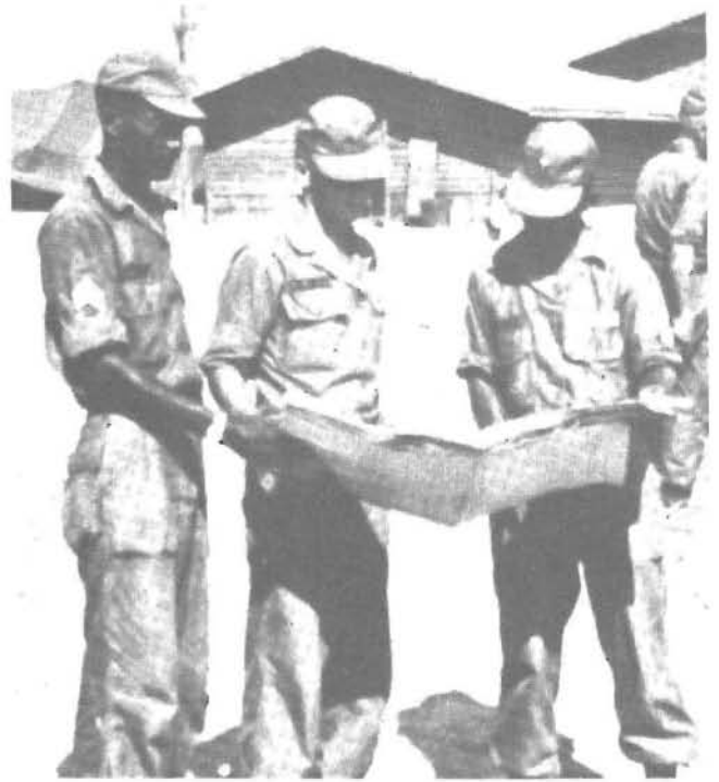
Engineer troops buiding hospital at Qui Nhon in 1966.
