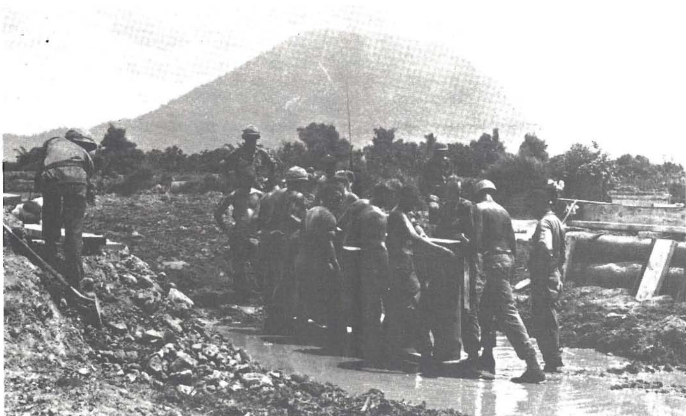
Engineer troops construct a bridge in the shadow of Nui Ba Din—the Black Virgin Mountain in Vietnam.
