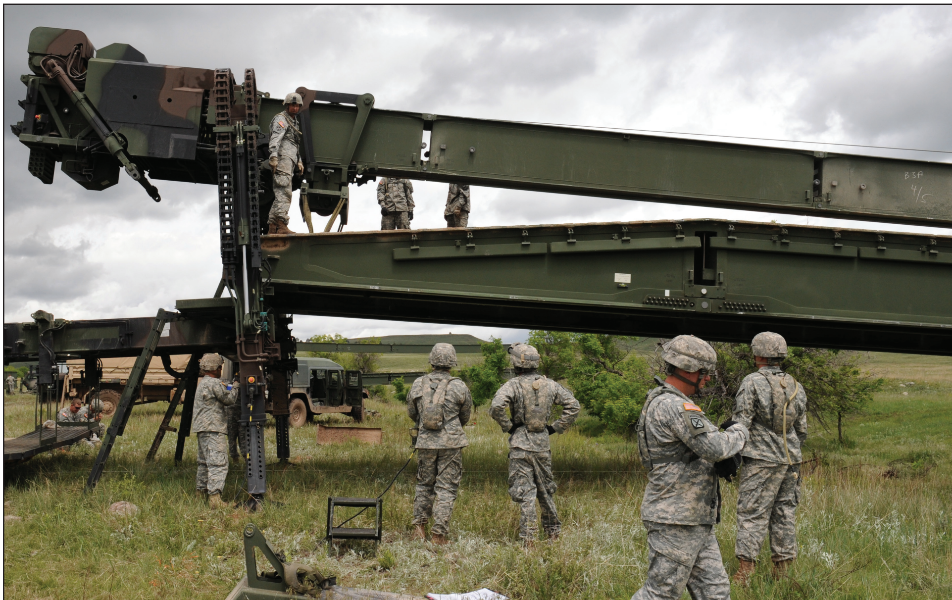
Members of Detachment 1, 200th Engineer Company out of Chamberlain, S.D. assemble a heavy dry span bridge during the 25th annual Golden Coyote training exercise in the Black Hills of South Dakota, 6-2 June.
