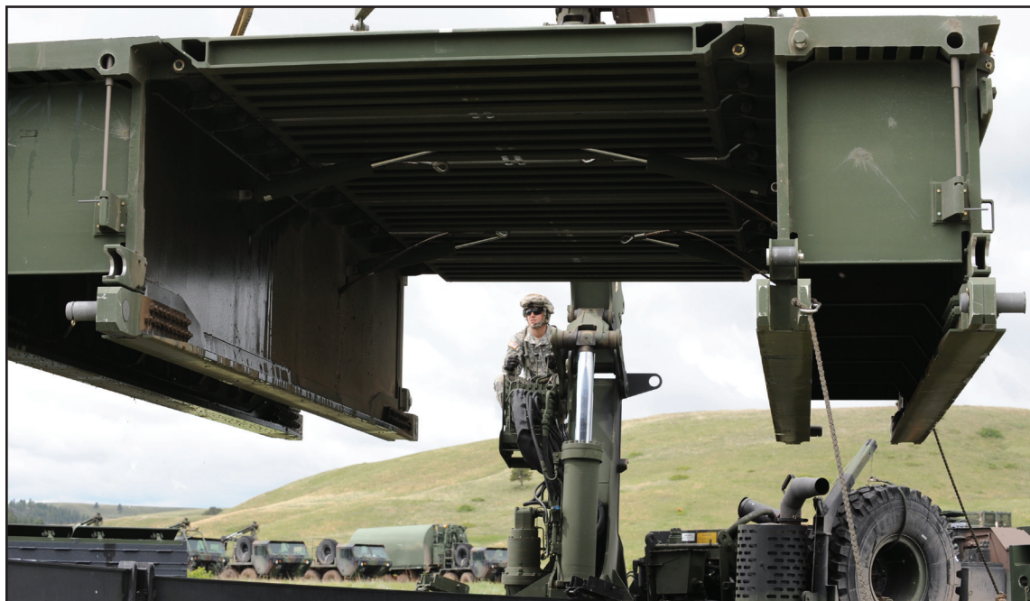
Above: Sgt. Martin Konechne, from Kimball, S.D., a bridge crewmember with Detachment 1, 200th Engineer Company in Chamberlain, S.D., operates a crane to lift a section of a heavy dry span bridge onto a bridge launch vehicle. Engineers with the 200th Eng. Co. maneuver equipment into place. Right: From left, Staff Sgt. Michael Dejong, operates the bridge’s launch vehicle as Sgt. 1st Class Dave Trautman Jr., supervises.
