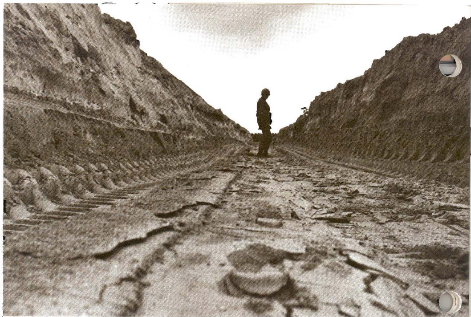
Cross-section of finished anti-tank ditch
