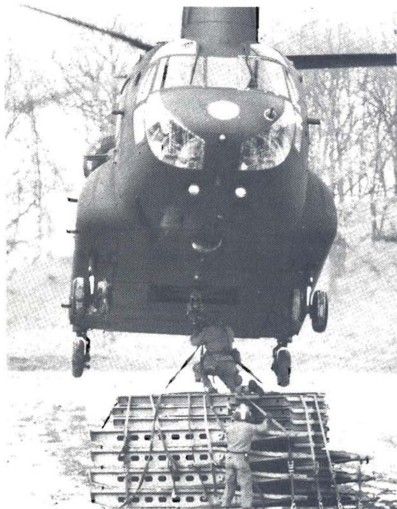
Chinook being hooked to MGB deck filler panels
