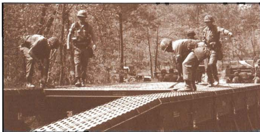
Above, equipment of the 27th Engineer Battalion (Combat) (ABN) is airdropped onto a DZ at Fort Bragg during ARTEP. Right, members of the 264th Engineer Company (MGB), Composite Battalion, emplace panels of the Medium Girder Bridge during recent training exercise
