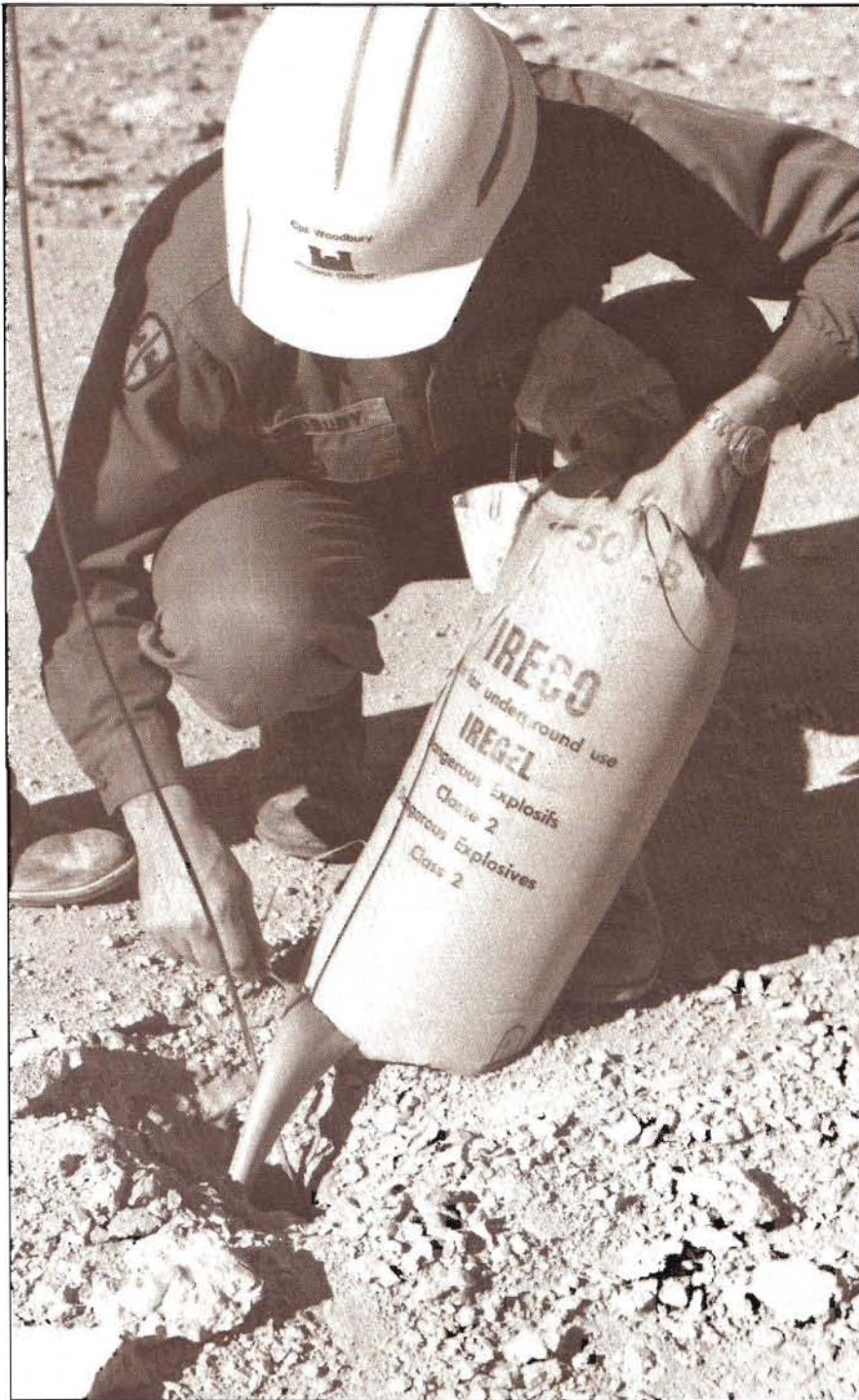
FIGURE 4 Pouring slurry into shaped charge blast hole
