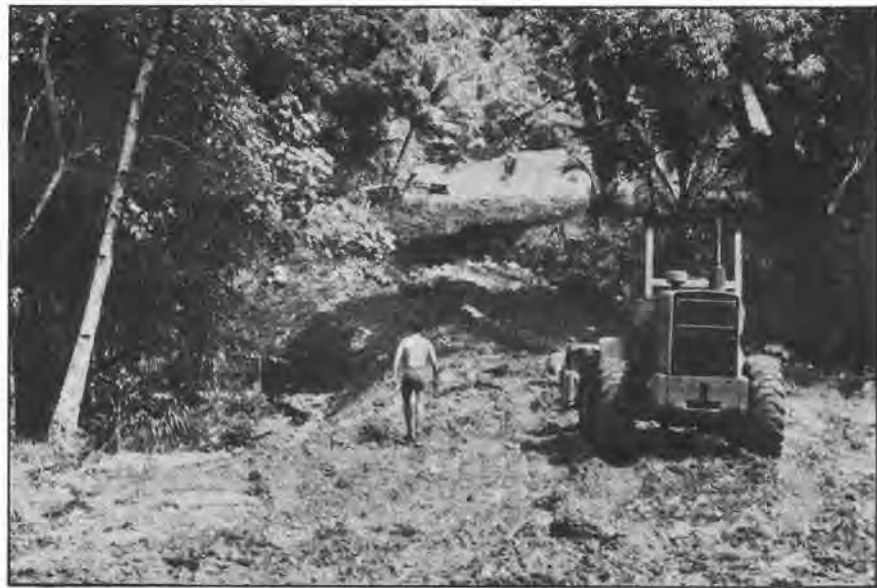
Starting road building operations through the jungles of Ponape.
