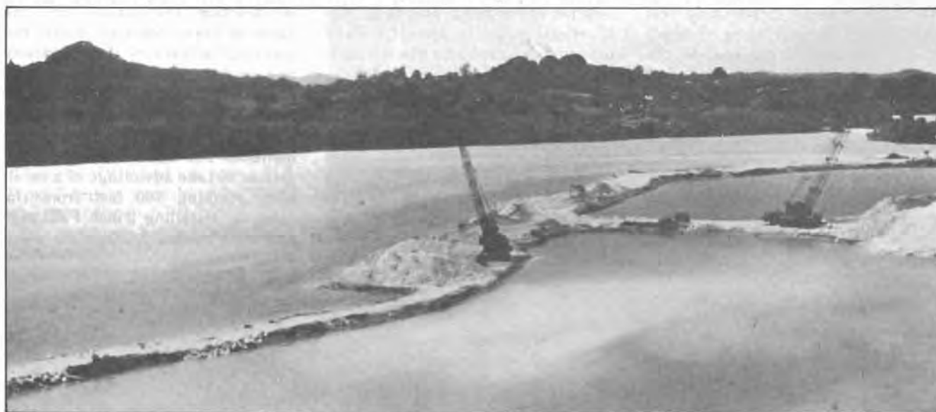
Coral dredging operations in Ponape. The coral was used as fill during road building projects.
