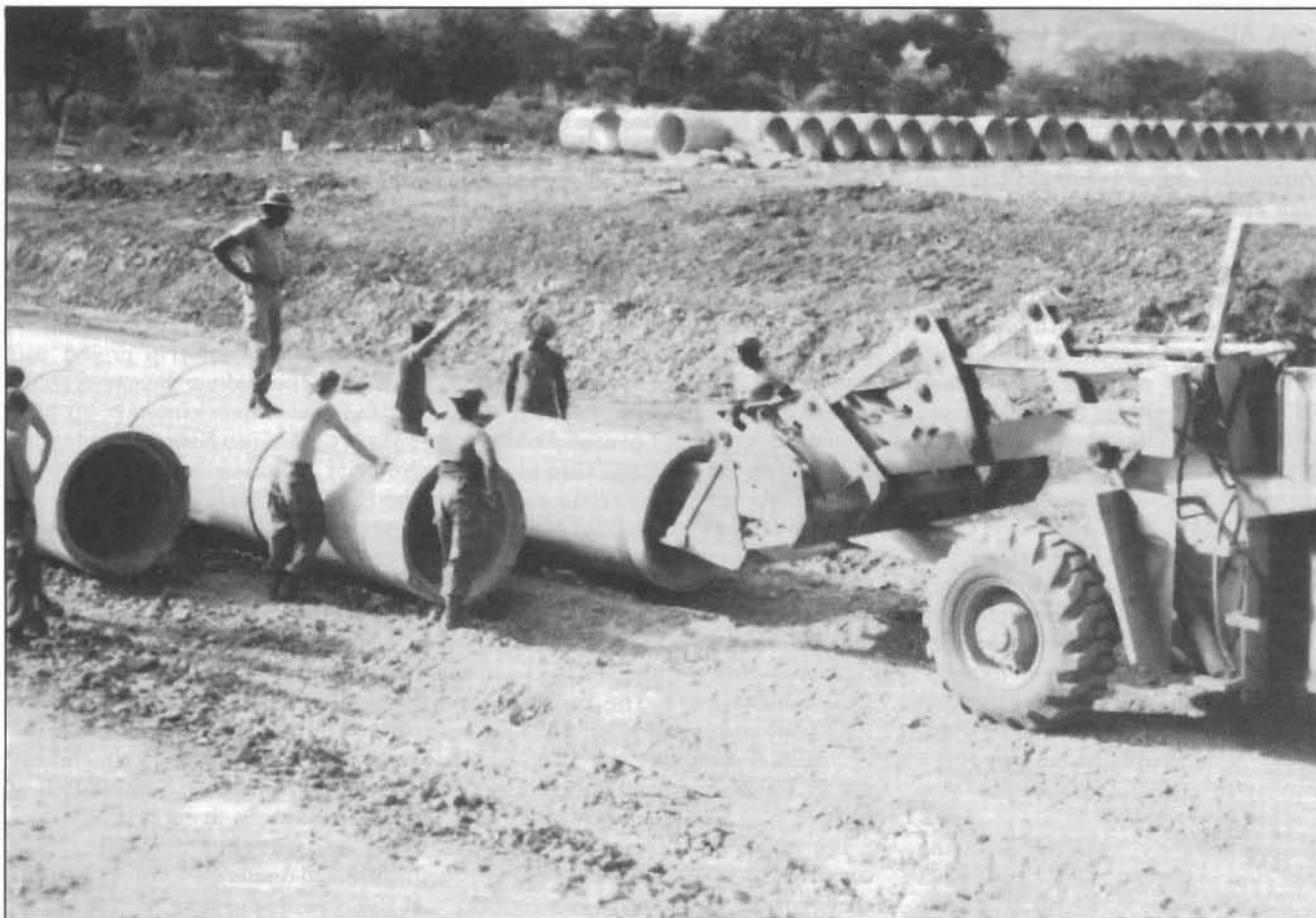
Engineers from the 46th Engineer Battalion install culvert sections at a triple-barrel site to carry runoff and stream water. To save time, materials, and money, the Engineers also constructed a trapezoidal channel to carry water from the runway (photo by 1LT Samuel Burkett).
