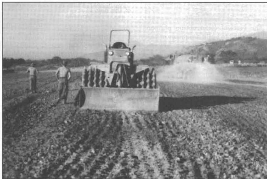
A high-speed compactor/motorized sheepsfoot roller was the most critical piece of Engineer construction equipment at the two airstrips in Honduras (photo by 1LT Samuel Burkett).
