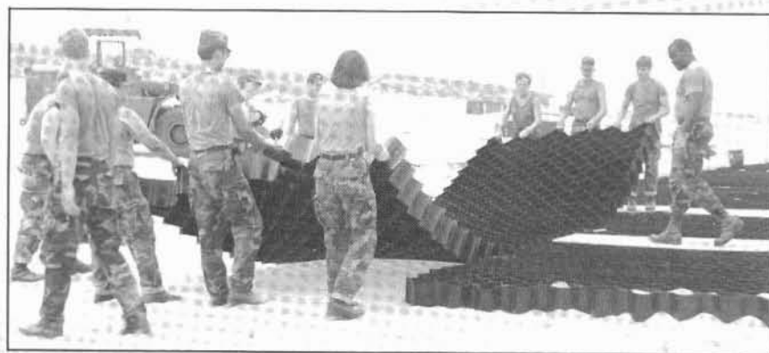
Sand grids are expanded and filled with sand. The 4-inch thick sections can be expanded to 20 feet and a light layer of liquid asphalt can be applied to provide a durable surface for wheeled traffic.
