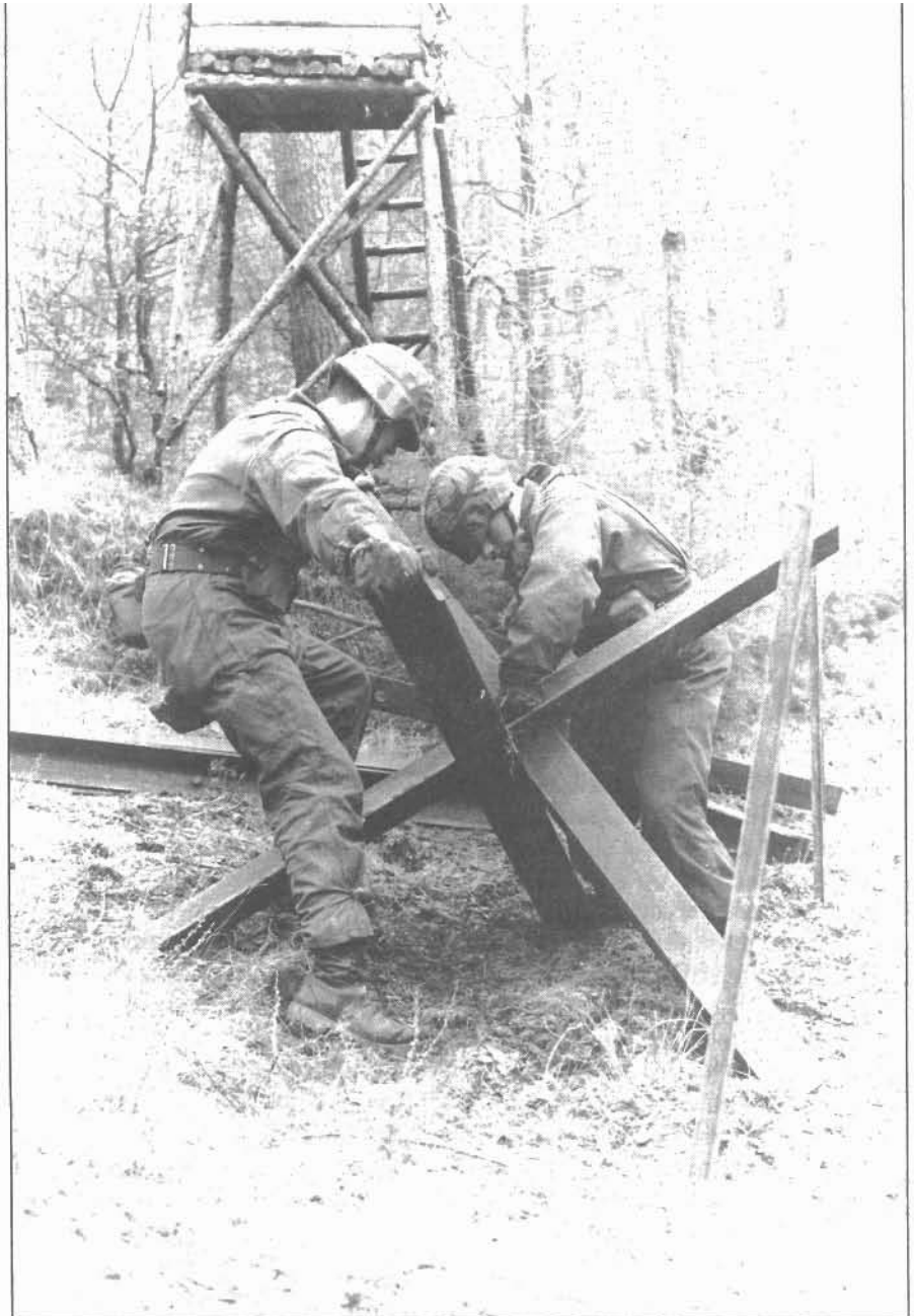
Combat engineers bolt together pieces of angle iron to form a hedgehog. While not designed for wartime use, hedgehogs serve as valuable training devices (U.S. Army photo).
