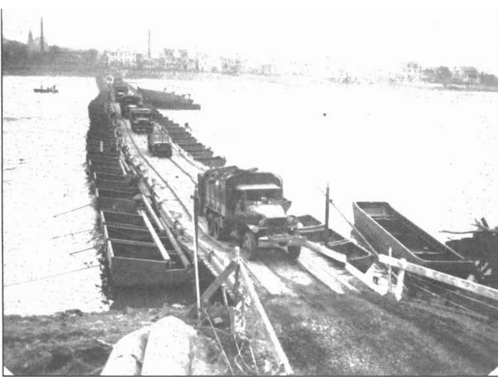
Traffic rolls over a heavy pontoon bridge built over the Rhine River at Kripp, Germany, in 1945. This was one of many bridges built by the 51st Engineer Combat Battalion during their march across Europe (U.S. Army photo).
