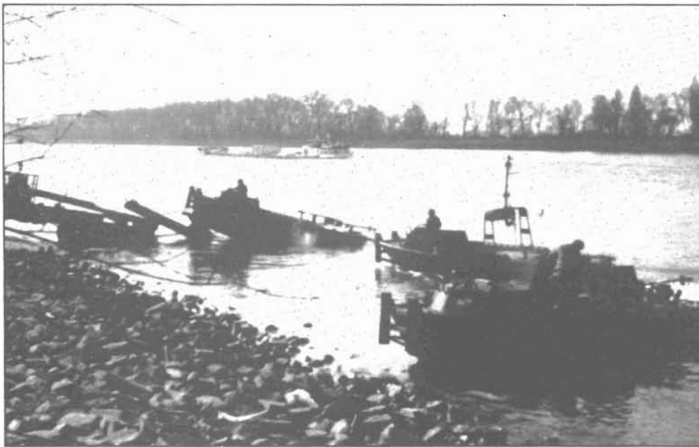
The safety boat should be the first craft launched during a bridging operation. A trained lifeguard should remain onboard this boat until all training is completed (U.S. Army photo).
