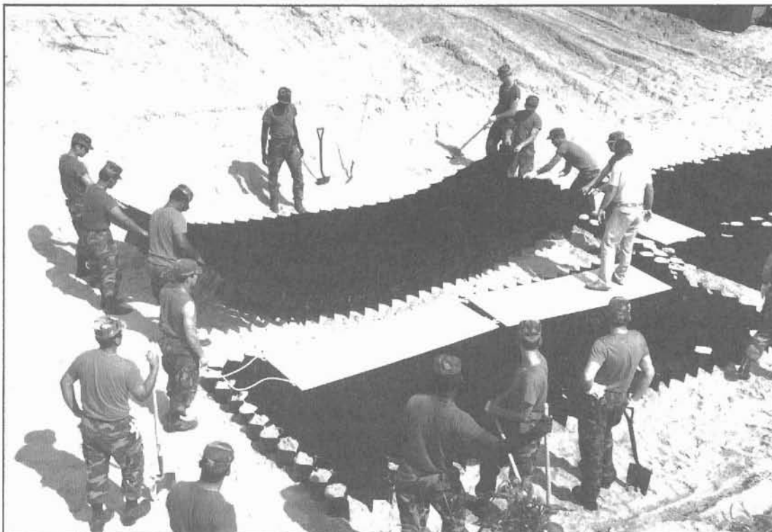
Road construction with sand grid proceeds quickly. Here, soldiers are expanding and emplacing sand-grid sections at Fort Story, Virginia.
