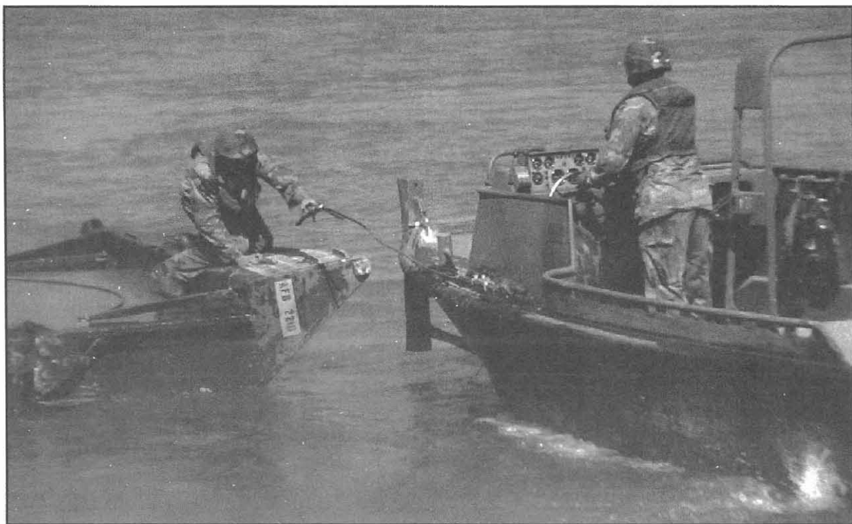
Engineer soldiers maneuver a bridge into position by hooking a boat to the bridge.
