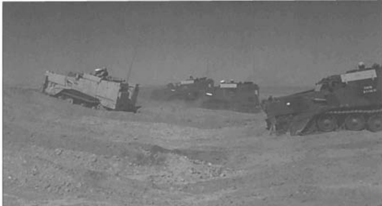
Soldiers of the 317th and 11th Engineers construct berms to improve force protection.
