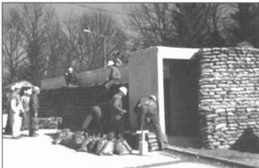
Multinational Division-North soldiers construct a 100-man bunker.
