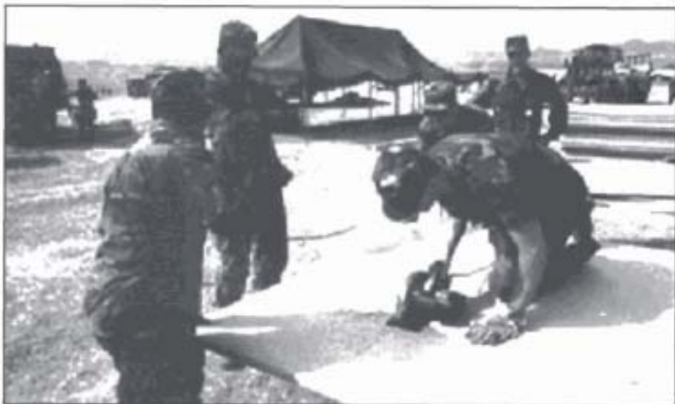
18th Engineer Brigade Construction, Operation Provide Comfort
