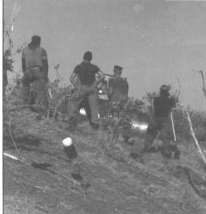
Engineers upgrade the obstacle belt in 1997.
