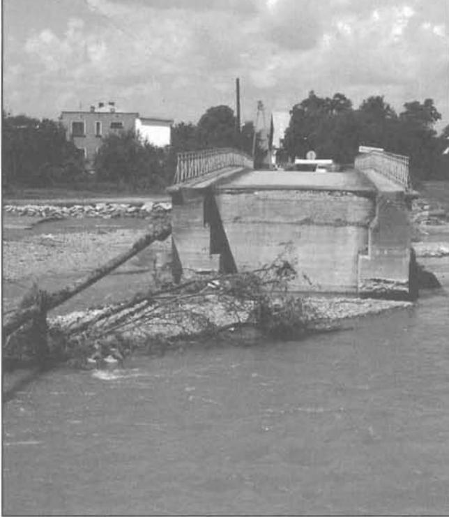
**Figure 2. A washed out embankment behind a bridgehead. A 60-meter section of the access road was destroyed (Bystrzyca Dolna town - Bystrzyca River).**
