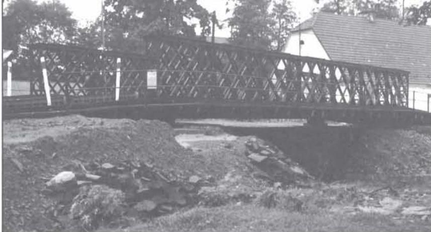
**Figure 4. Free-supported spans in a DMS-65 structure in the basic arrangement. It has a 21-meter span with 6-meter entry spans stretching  $L_c = 7$  meters (Roztoki - Miedzylesie Commune on the Nysa Klodzka River).**
