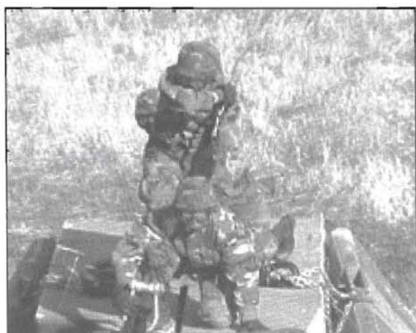
Soldiers from the 814th Engineer Company prepare to hook a ramp bay.
