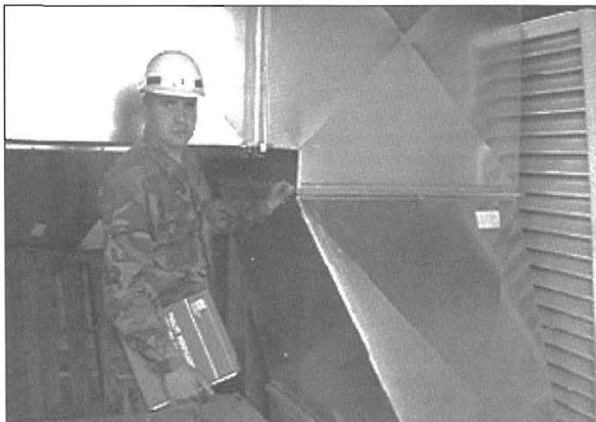
1LT Jeff Qualteri served his internship at the Portland District's Bonneville Lock and Dam. He is shown inspecting recently installed ductwork.
