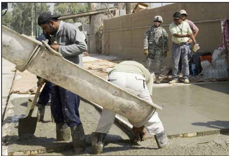
Photo by Lt. Col. Rhonda McGuire, JASG Public Affairs Staff Sgt. Christina Matlock (center) supervises as local contractors smooth a section of wet concrete shortly after pouring it into a form. Matlock supervises many of the concrete construction project in the IZ.
