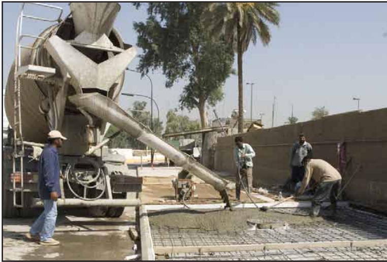
Photo by Lt. Col. Rhonda McGuire, JASG Public Affairs Local contractors pour and spread concrete into a form during a sidewalk construction project in the International Zone.
