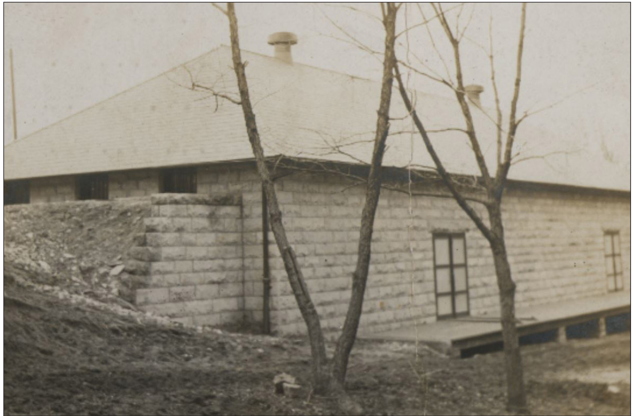
Courtesy photos Building 309 Holbrook Avenue, between Carter and Dickman Avenues, was built in 1906. Constructed from native limestone bldg. 309 was first used as a vegetable storehouse. This area of Main Post between and to the south of the Cavalry and Artillery Posts is referred to in historic terms by the Army Corps of Engineers as the Quartermaster Supply Service District. The buildings in this area served their respective functions in support of both posts. Today, building 309 is being used for storage.
